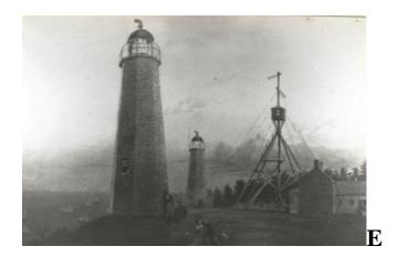
The agent would then move a dial with the numbers 1 to 10 and the words "look out" and "repeat." If he dialed a number from 1 to 6, the upper arm on the semaphore above the shack's roof would move to the corresponding number. If he dialed 7 to 10 or either word, the lower arm would move correspondingly.
